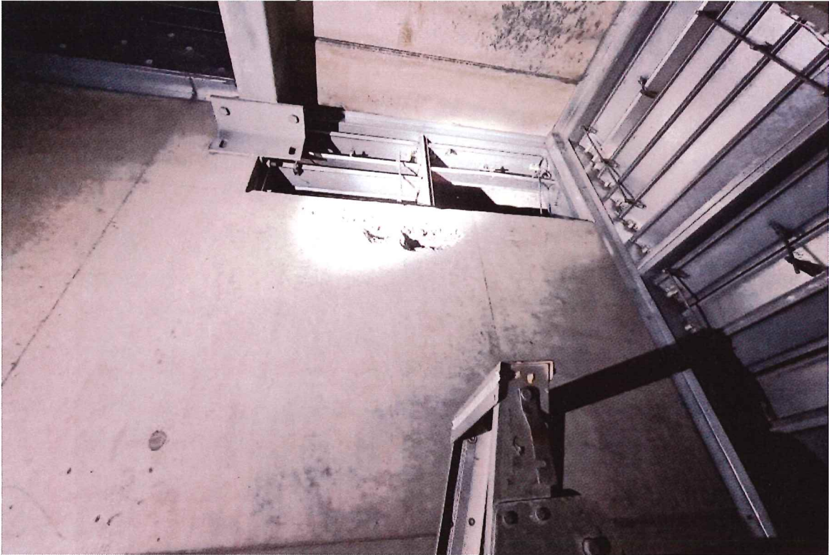
1.4 Multiple exit points through metal cladding and ventilation mesh. Note marking on ceiling from repeated strikes.
